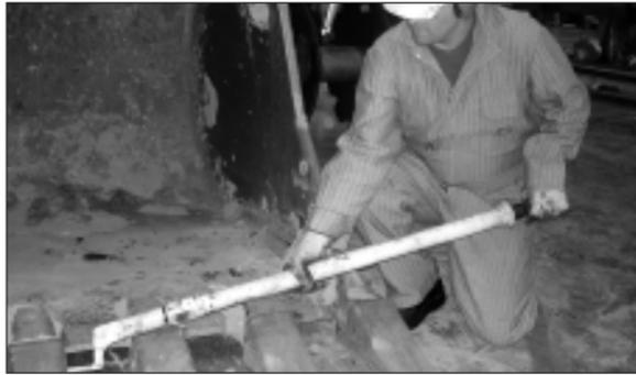
5. Thrust the drive bar forward to knock out the pin. The amount of force required to drive out each pin varies with the amount of corrosion/foreign matter on the pin and other factors. Always start with lighter force to gauge the pins movement before taking a full swing. Multiple strikes may be required.
