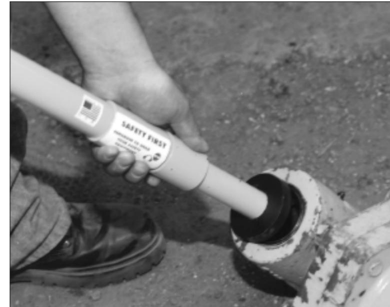
1. Select the proper driver adapter and attach to the plunger of the Slide Sledge™ Multi-Head™
